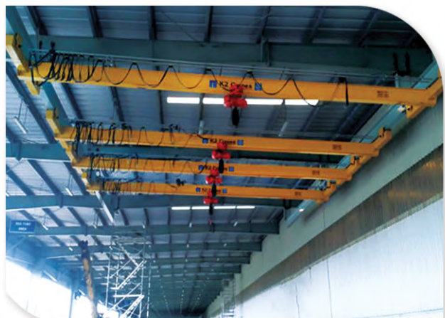
UNDERSLUNG CRANE CAPACITY: Up to 5 ton
